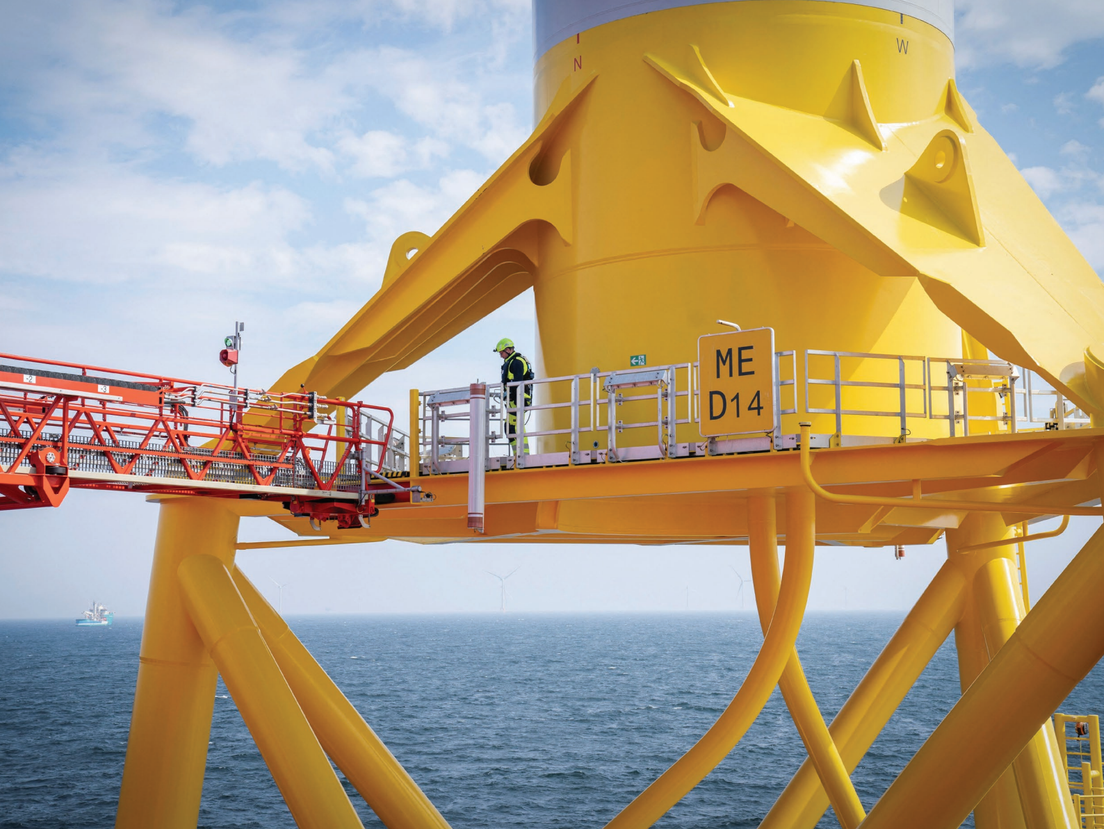
The 'walk to work' gantry of the Esvagt Alba ship is connected to a turbine at the Moray Offshore Windfarm East, off the Aberdeenshire coast in August 2021. Photo: Jane Barlow / Getty Images
